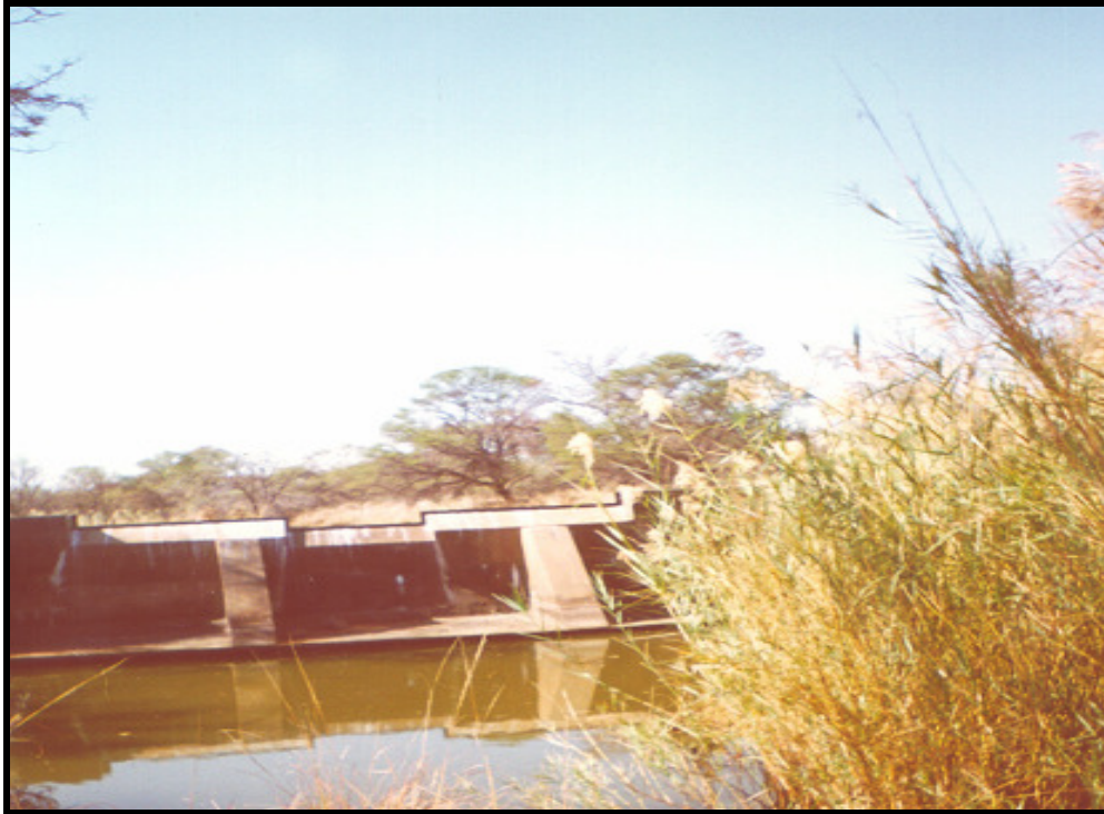
Figure 2.8 (a) A dam just above the Tobias site.
