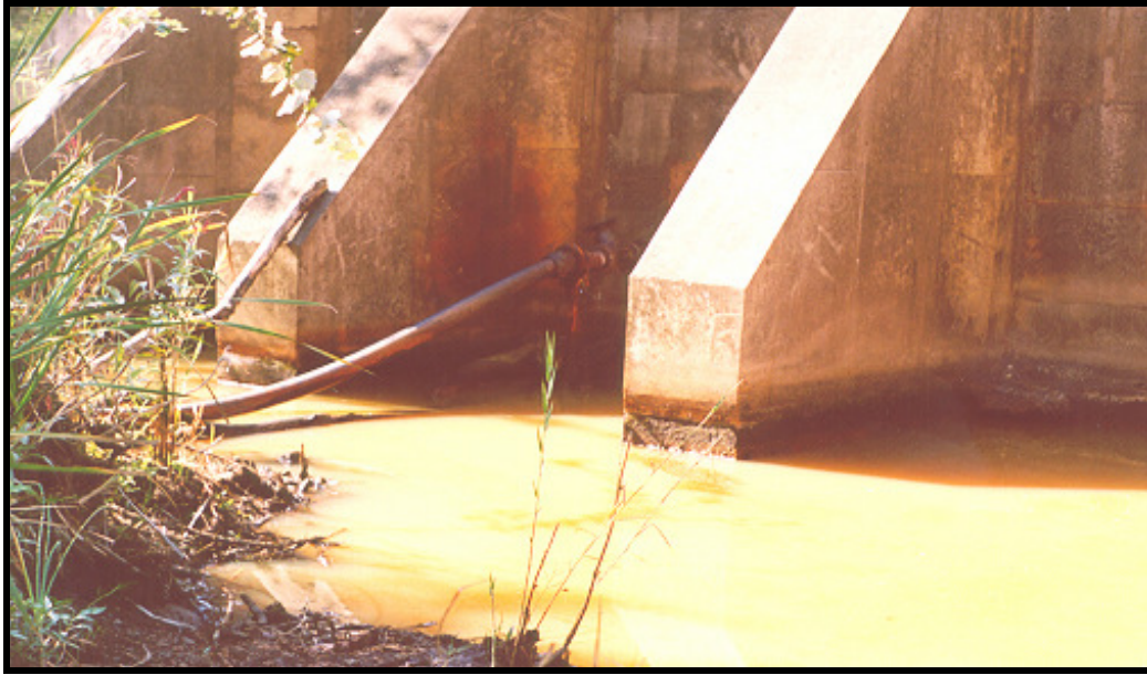
Figure 2.5 A dam on the Naboom Spruit at the Mine site.
