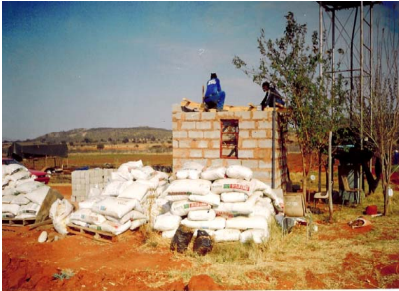
Bags of manure near the still being constructed office cum storeroom
