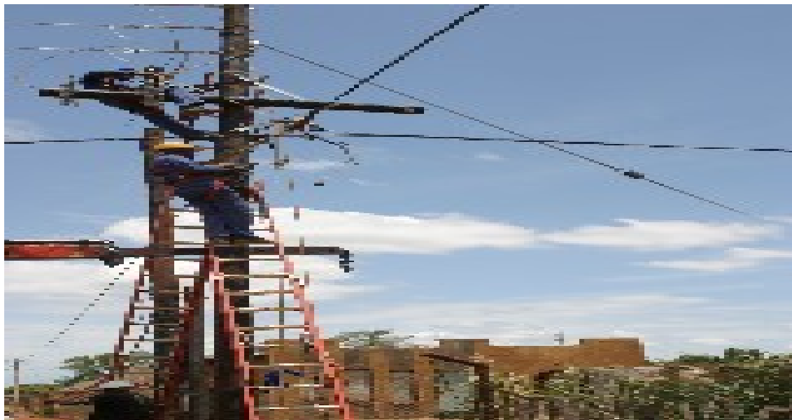
Picture 5: Muyexe Electrification Project
