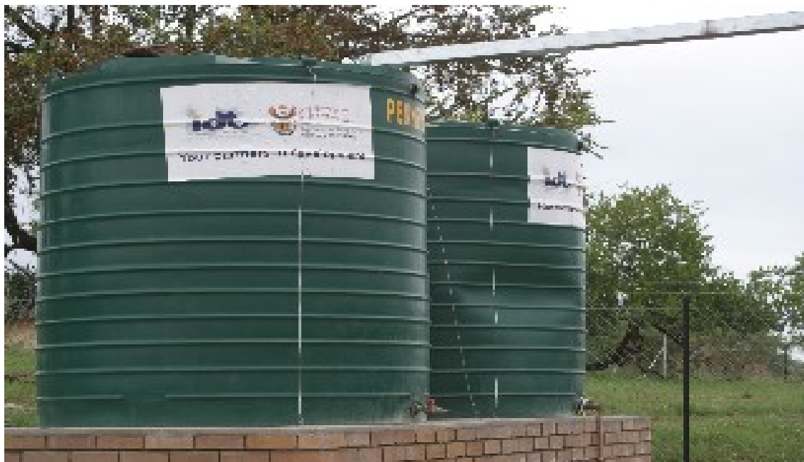
Picture 9: Water tanks distributed to all families
