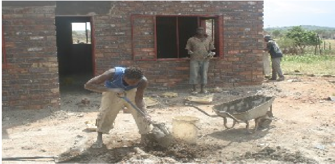
Picture 3: Housing Project in progress in Muyexe
