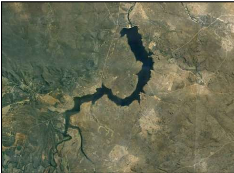
Figure 2.2: Aerial view of Flag Boshielo Dam, Limpopo Province, South Africa (Adapted from https://www.google.com ).
