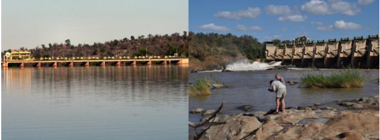
Figure 1.3: The sluices/gates of Phalaborwa Barrage.
