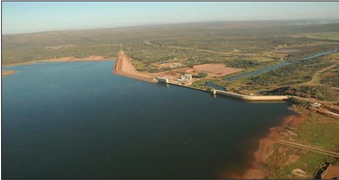
Figure 2.3: Dam wall of Flag Boshielo Dam ( http://www.DWAF.gov.za ).
