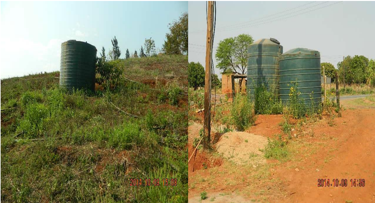
Photograph 10: Water Storage Tanks for Crops and Vegetables Irrigation
