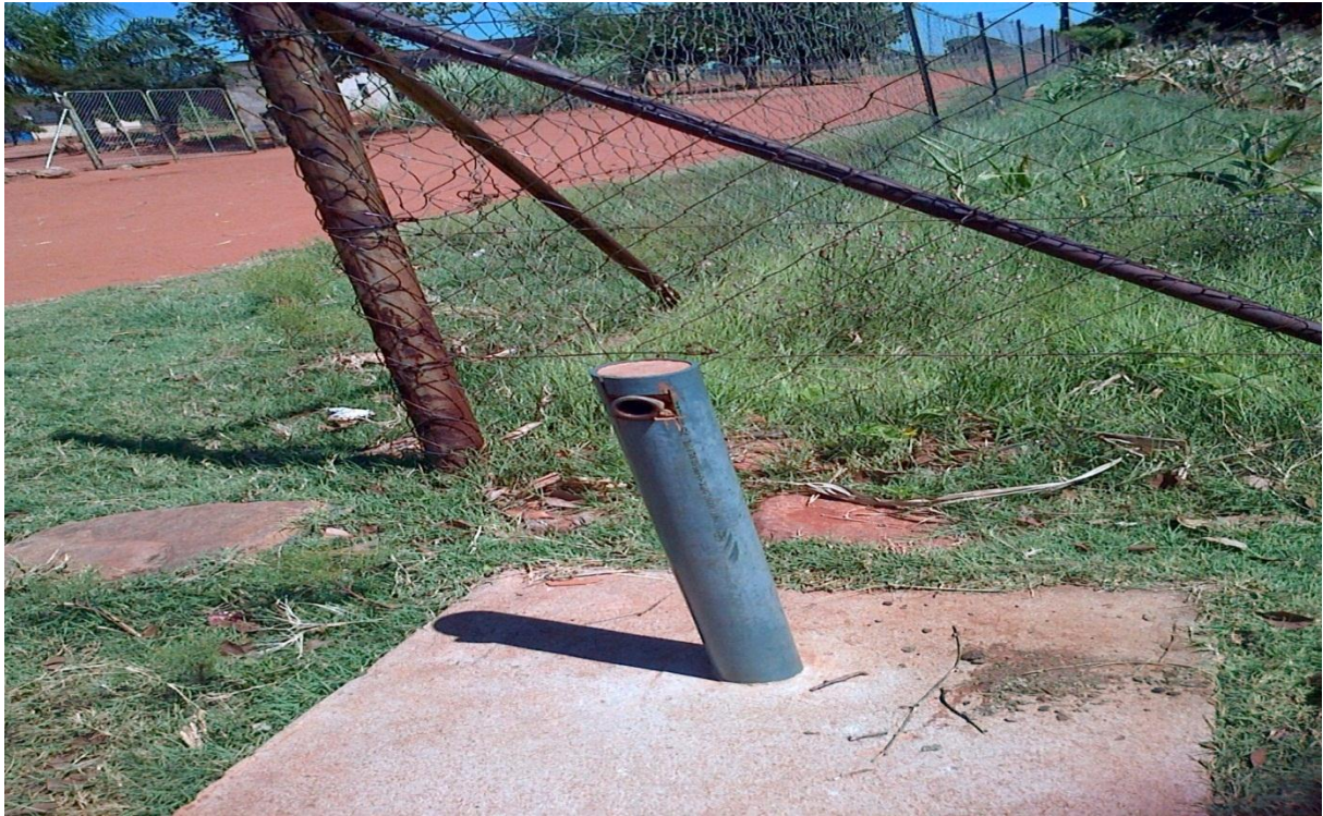
Figure 17: Broken tap
