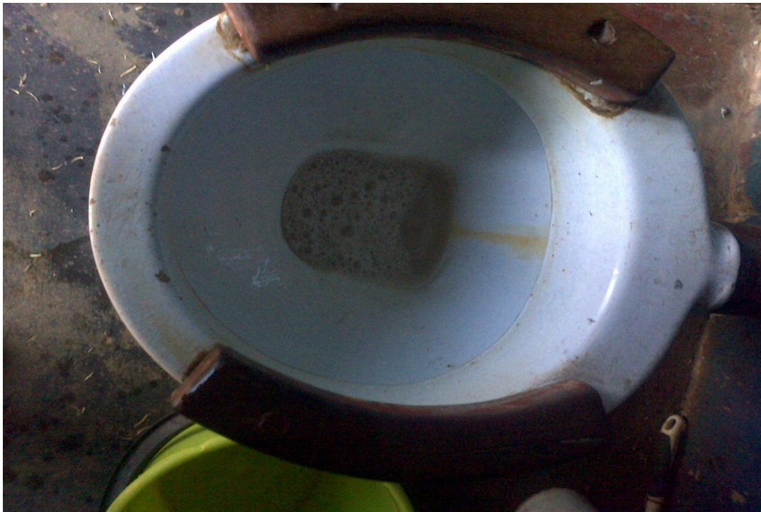
Figure 26: Toilet flushing with greywater
