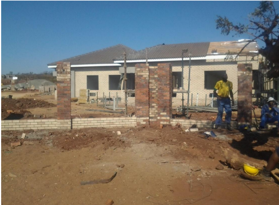
Picture 4: Muyexe police station under construction.
