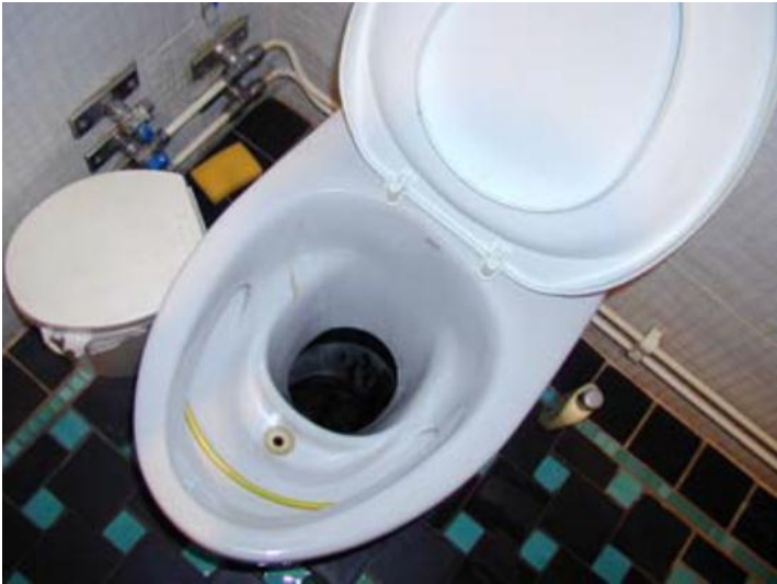
Figure 2.5: UDD toilet (Source: EcoSanRes, 2008)
