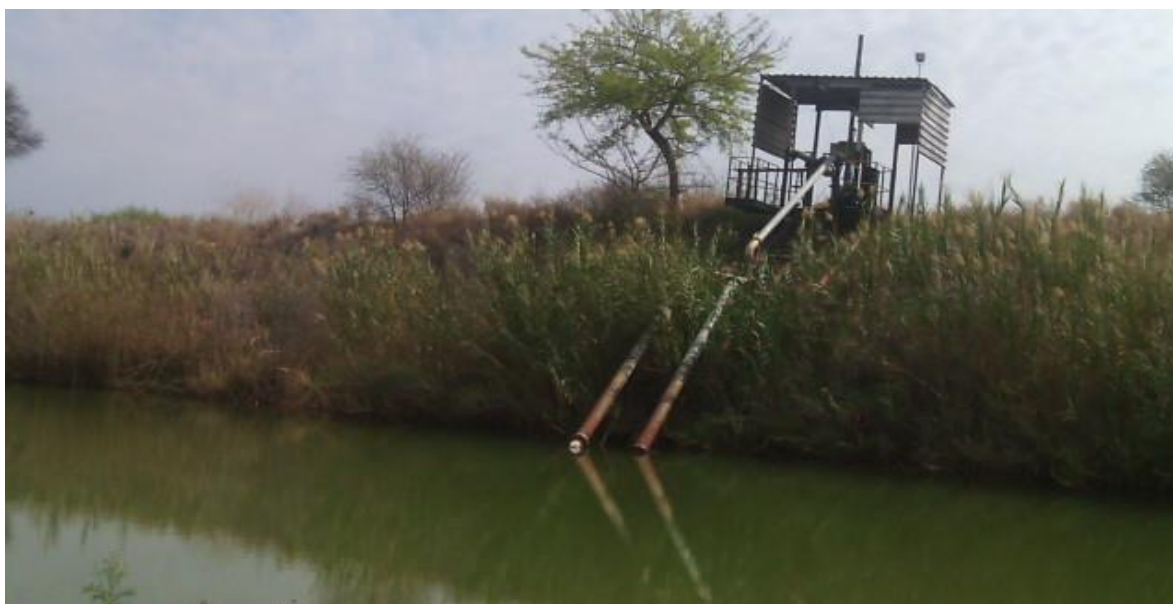
Figure 3.7: Photo depicting water abstraction system in Mokolo River for irrigation purpose
