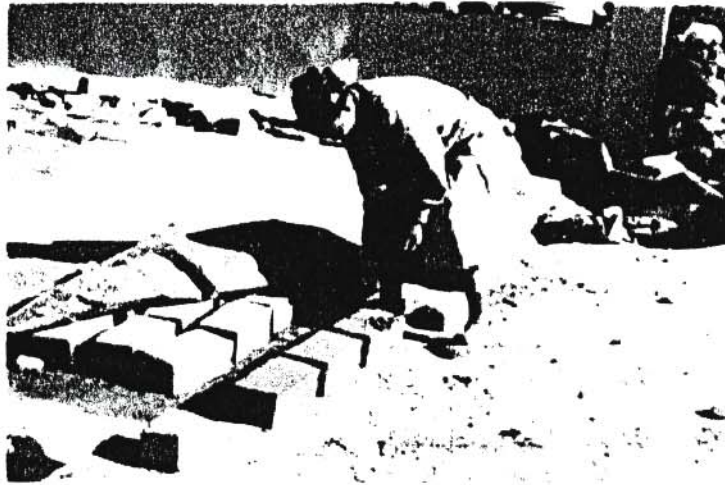
FIGURE 3: PHOTOGRAPH- SOIL CEMENT BRICKS
