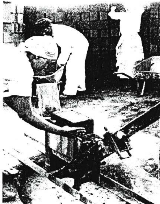
FIGURE 2: PHOTOGRAPH- SOIL-CEMENT BRICK MANUFACTURING
