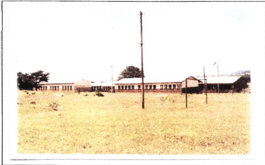
KOLOBETONA SENIOR SECONDARY SCHOOL
