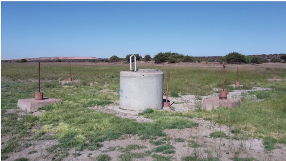
Figure 1. Borehole infrastructure of the aquifer recharge program at the Postmasburg dryland floodplain.
