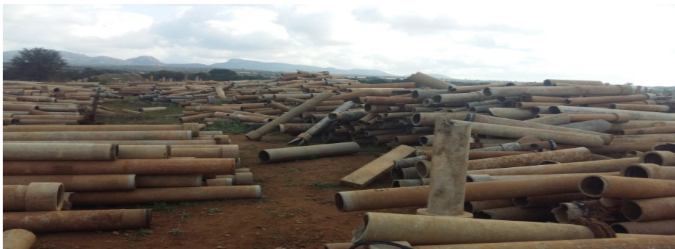
Figure 2.4. Temporary storage of asbestos pipes in Modjadjiskloof
