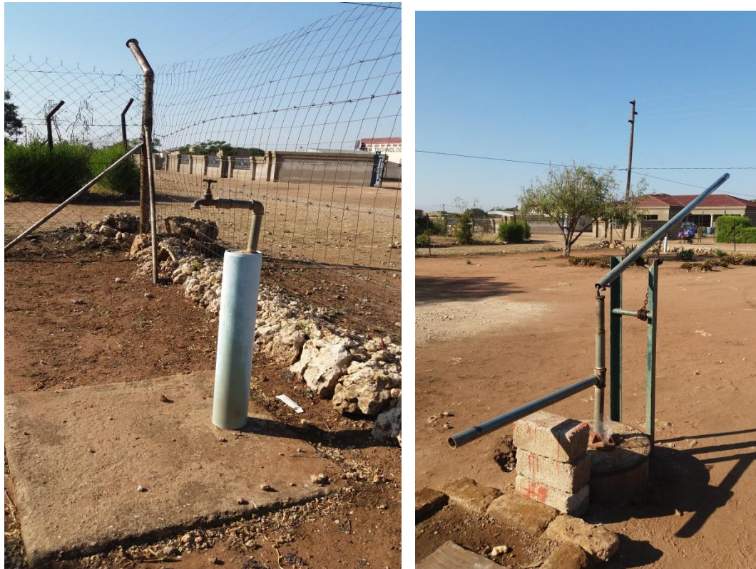
Figure 4.6: An illustration of standpipes in the yard and boreholes
