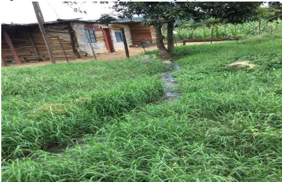
Figure 3.1: Picture showing open sewage pipe flow in front of the house
