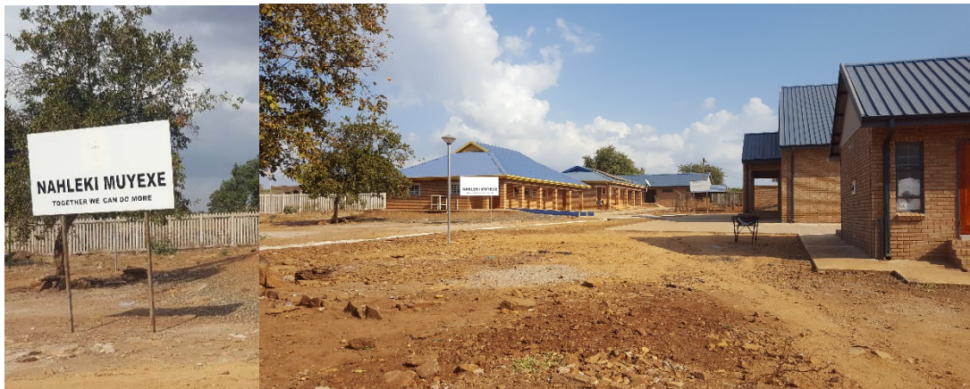
Figure 4.7. Nahleki Muyexe centre: Muyexe village was provided with the Hlaneki Muyexe Community Centre which was provided by using the Comprehensive Rural Development Programme. The centre consists of the community market, community hall, post office, computer centre and the Thusong service centre. The post office and the women’s self-help are the only facilities in this centre which are operating, it is not known as to when will the other facilities start to operate. The closure of these facilities have promoted lack of employment to women in Muyexe village.
