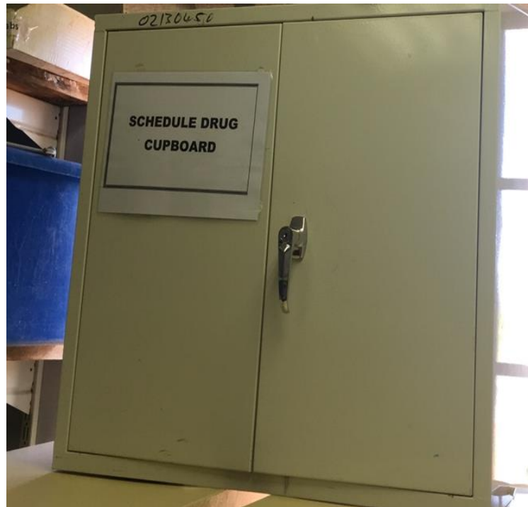
Figure 4.4: Schedule 5 cupboard in clinic C
