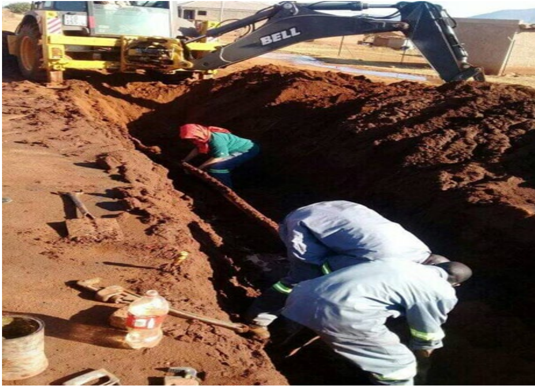
Figure 4 Municipal officials doing maintenance of the old pipes
