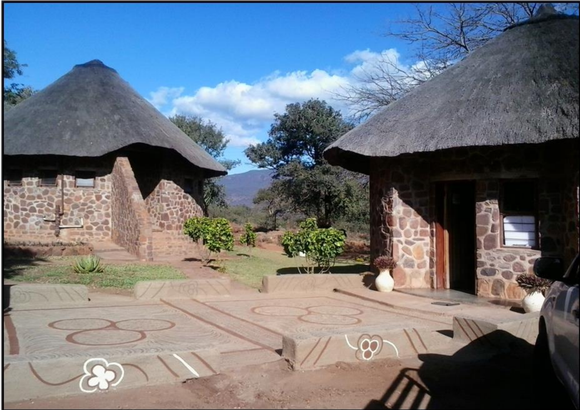
Figure 5.4. The current condition of the Dzata Provincial Heritage Site.
