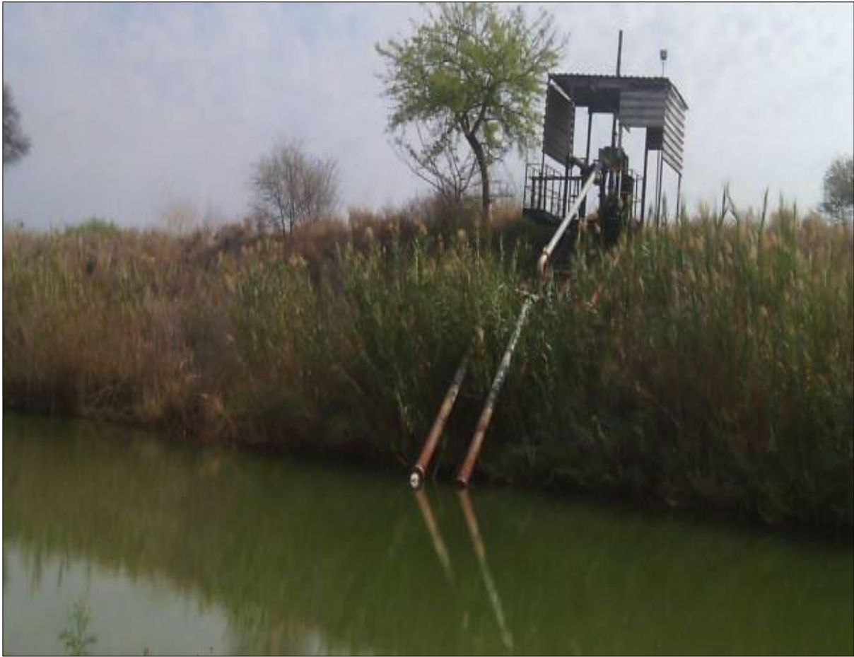
Figure 3.5: A photo depicting water abstraction system in Mokolo River for irrigation purpose
