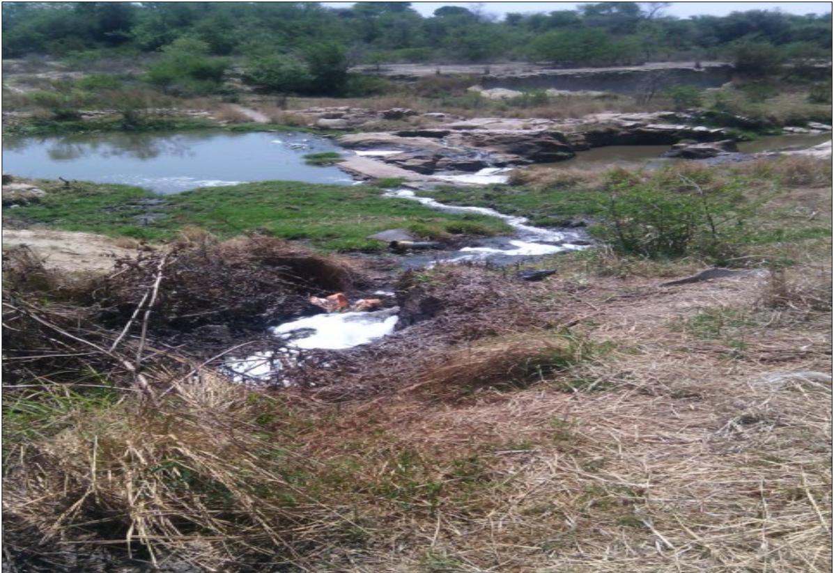
Figure 3.3: Untreated sewage waste flowing into the River
