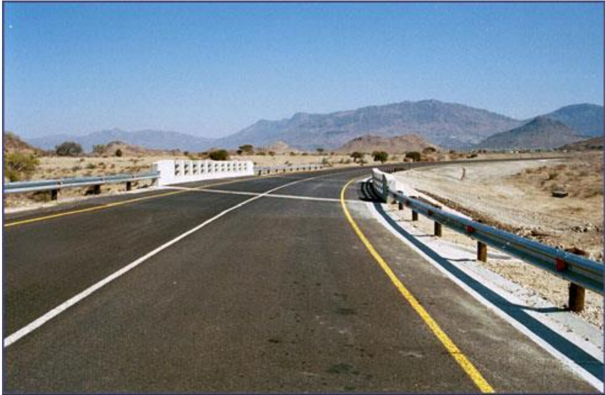
Figure 4.15: Road construction by MPM (Implats, 2004)
