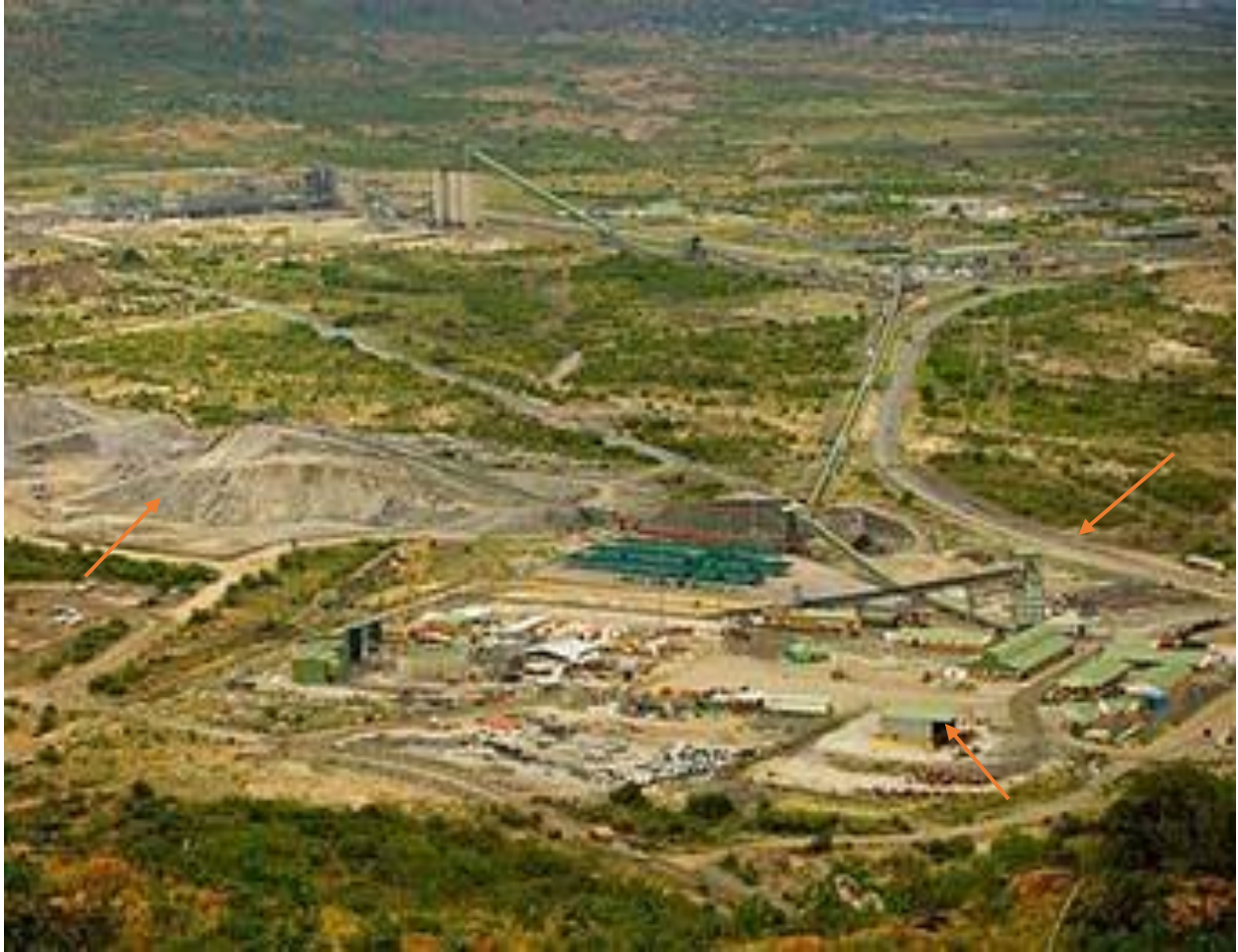
Figure 4.13: Land clearance for the establishment of MPM facility (Thovhakale, 2015)
