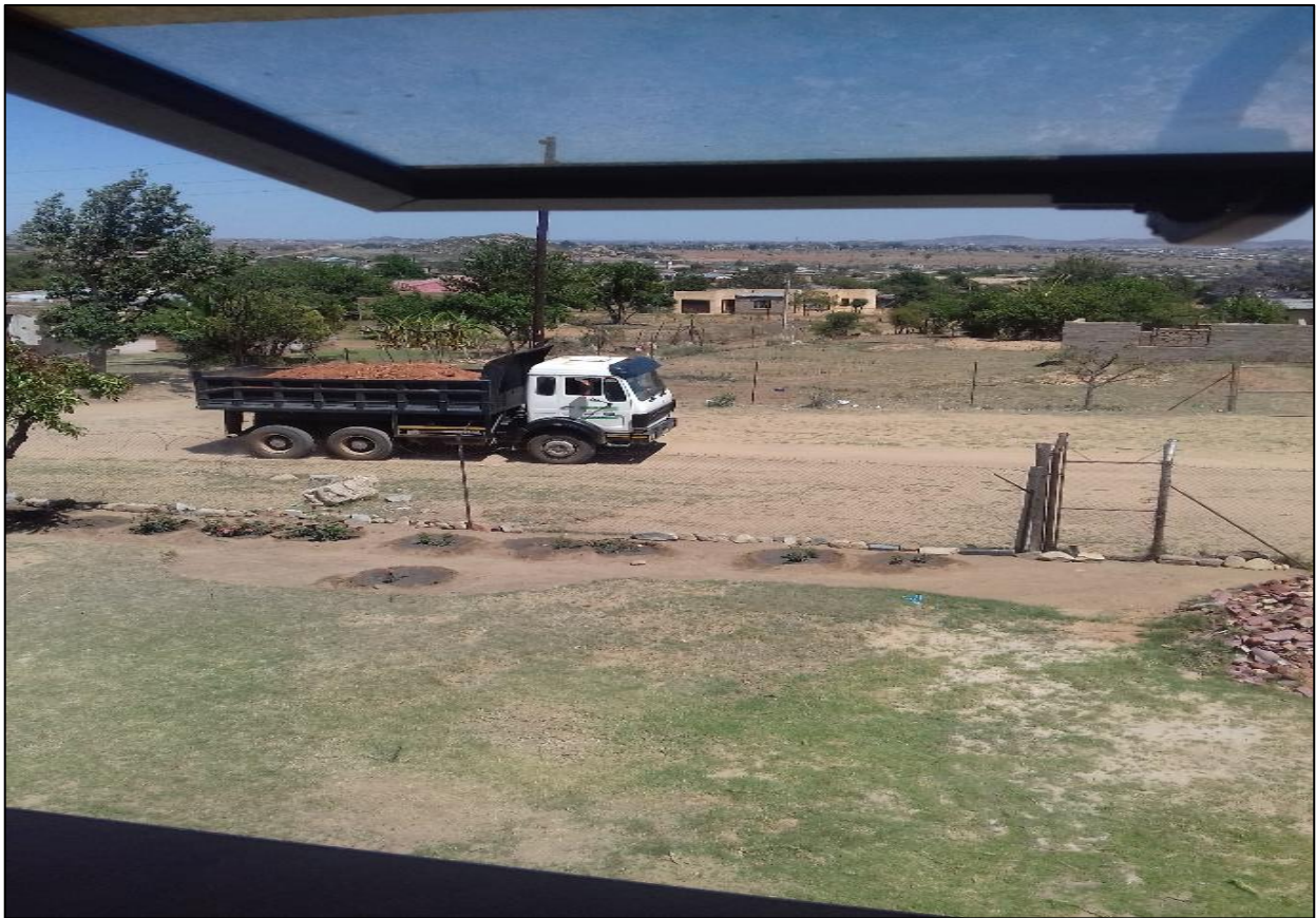
Image 2: Sand mining activities at Mentz Village
