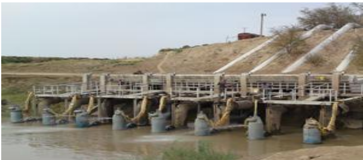
Figure 3.4 Example of Pumped surface irrigation system
