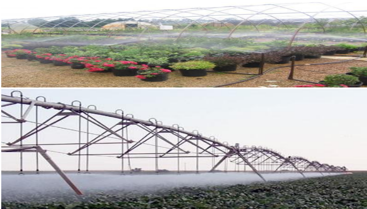
Figure 3.1 Example of overhead irrigation system
