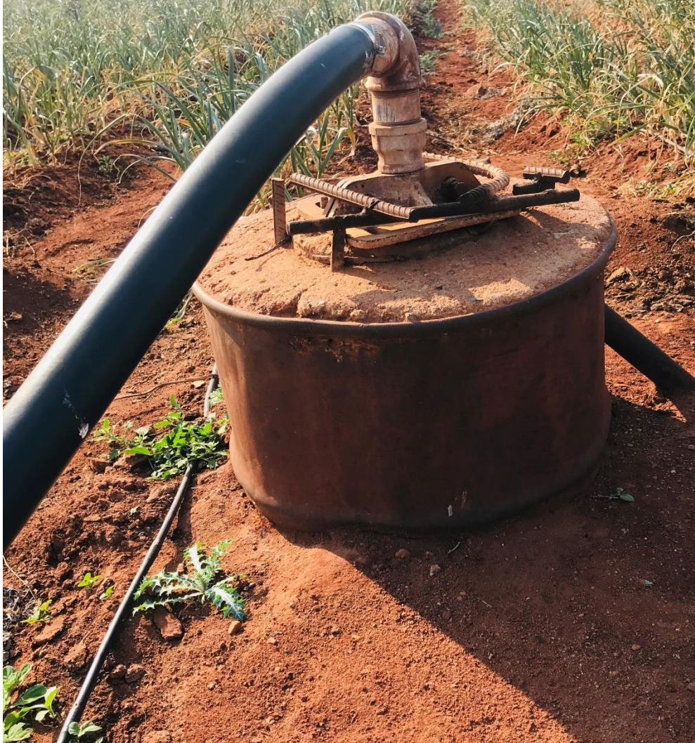
Figure 4. 2: Above ground borehole structure of the farmer
