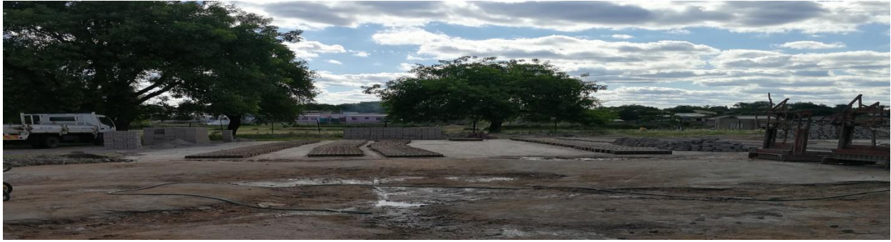
Figure 4.5 Manual machines, truck and bricks at Titirheleni Vamanana Brick Laying project
