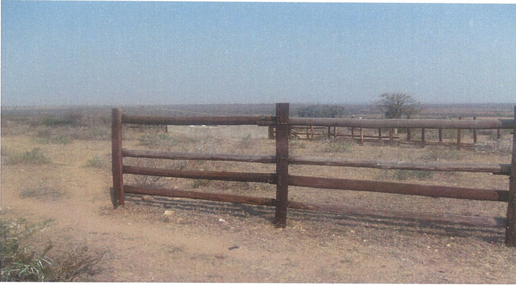
Pic.2 (dipping tank at Botlokwa Ramokgopa)
